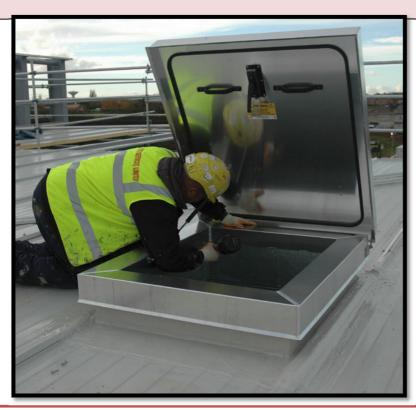
Quantum BS1 is the Rolls Royce of access hatches a bespoke, low profile aluminium unit, designed for mounting onto all types of flat roof, especially aluminium and steel standing-seam roofs.
