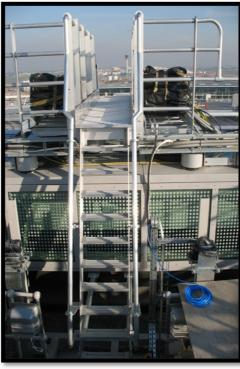
Quantum ships Ladders are a proven, all aluminium fully welded and tested ladder system. Manufactured in accordance with BSEN 516 system, it attaches to and compliments the Quantum walkway systems. This product allows specifiers to provide lightweight yet durable roof access for maintenance purposes on any roofing system. Each system is designed and tailor made to suit each project
